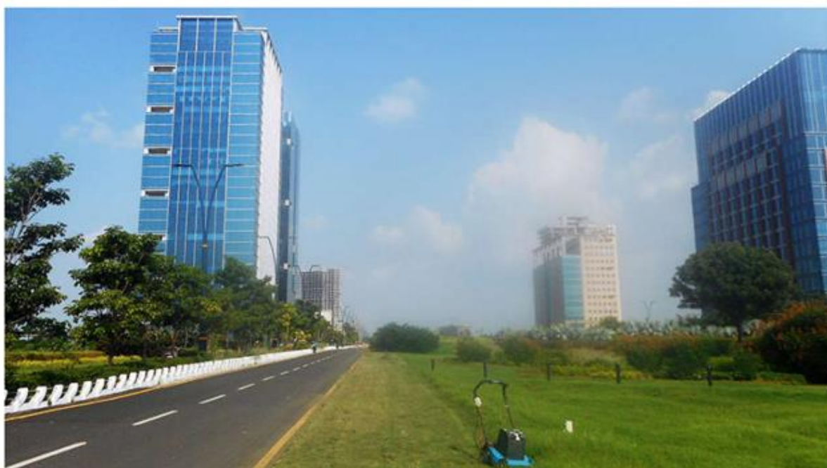
The towers on the left fall in the domestic-tariff area while those across the road are in the IFSC area. Together, they account for 9,000 jobs today at the Gujarat International Finance Tec-City near Ahmedabad; courtesy of N Sundaresha Subramanian
